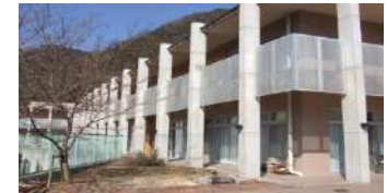
Fukayaso,Nursing Home in Okayama
