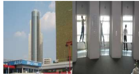
Elevator in Sumida city Hall ,Tokyo
