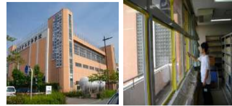
Tokyo Gakkan Niigata high school
