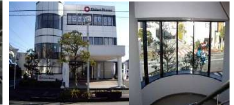
Daiwa house company
