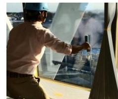
Apply vertically from the top on both sides to the center with little pressure. Do not stop the application on the center. Gradually apply lightly.
