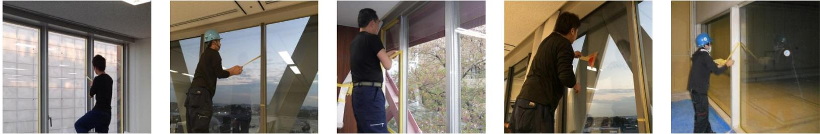
One hour after the application, touch the masking tape and confirm the liquid did not remain your fingers. Take off the masking tape carefully with both hands.
