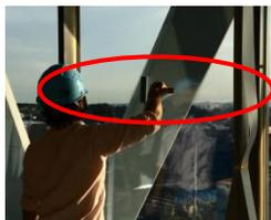
Apply over the joint line in parallel with little pressure.(40%)
