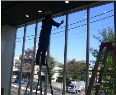
Ex) h3800mm\*w1200mm ※Divide the applied area if the glass is over h2500mm.
